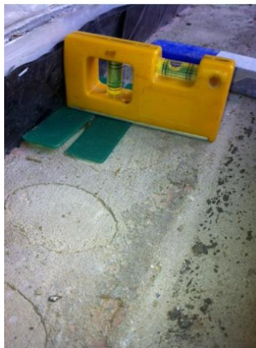
Photo 1 Levelling & packing front to back
