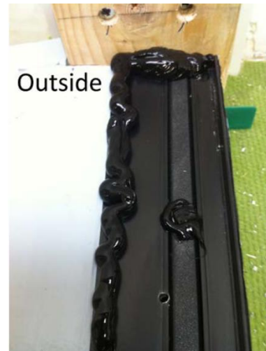
Photo 4 Silicone bead between sill and track
