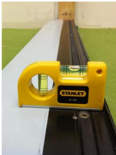
Photo 3 Checking sill is level
