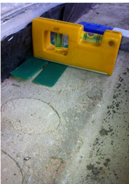
Photo 1: Levelling & packing front to back
