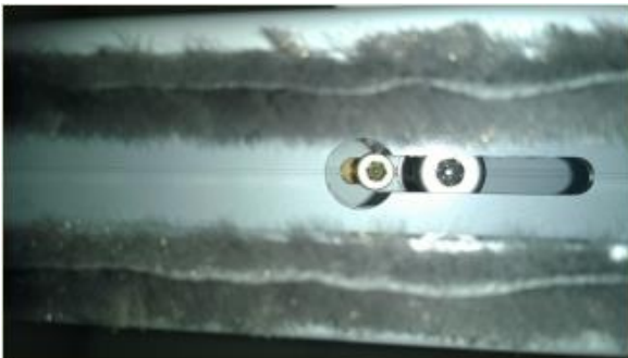
Top track fixing point, with adjustment screw on right.
