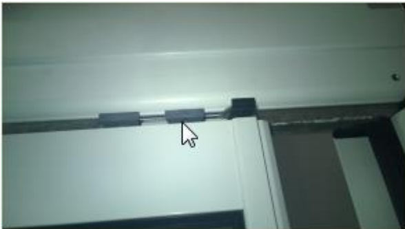
Locking lever turned 180° to cut-out side of top track .
