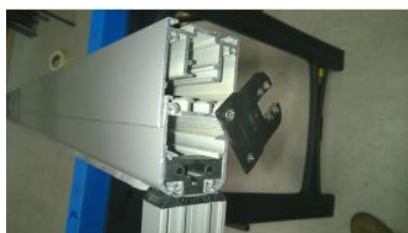
Side Jamb connected to top track.
