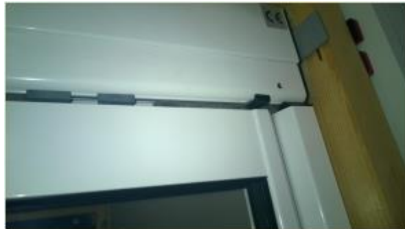
Lead panel pushed up to side jamb , Locking lever now has to be turned 90° away from the side jamb
