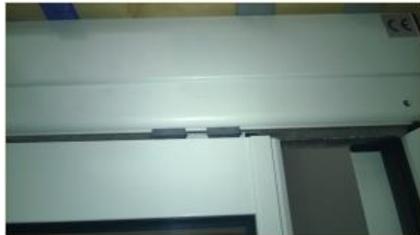
pivot wheel passed the Top track Panel locaters
