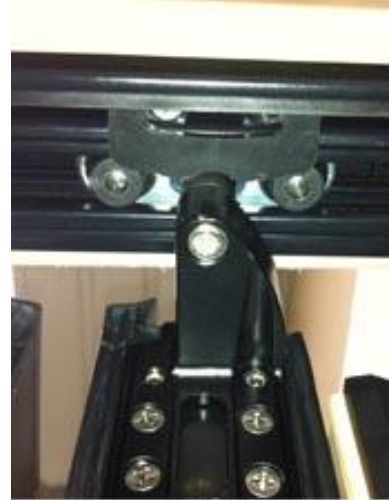
Photo 18 – completed stacking catch
