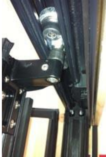
Photo 17 – adjustment bolt with collar
