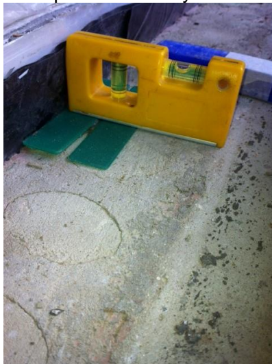
Photo 1: Levelling & packing front to back
