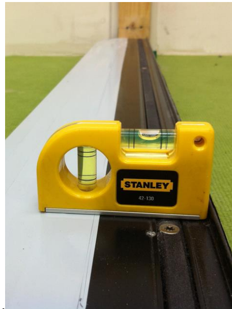
Photo 4 Checking sill is level
