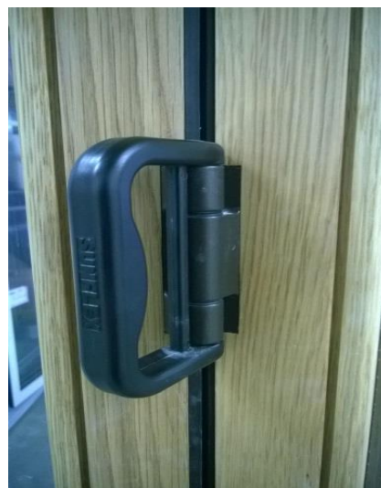
Photo 9 – fitted pull handle to outward opening systems
