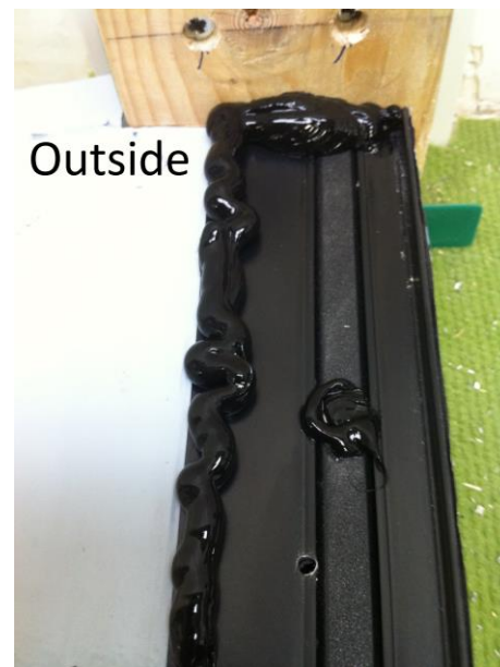
Photo 8 – Silicone bead between sill and track
