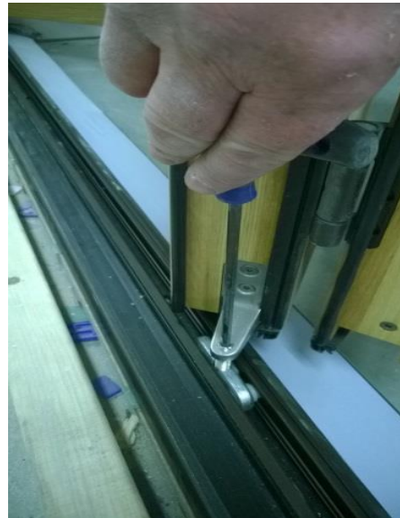
Photo 10 – Adjusting the setup height
