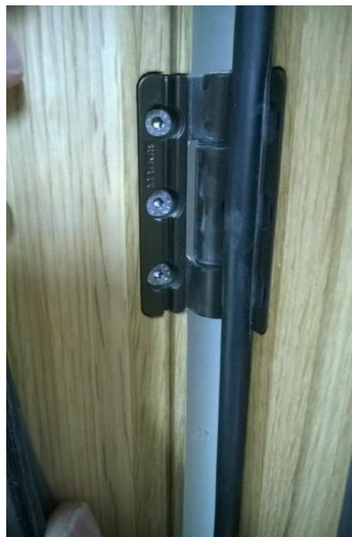
Photo 5 - Pre-drilled fixing location
