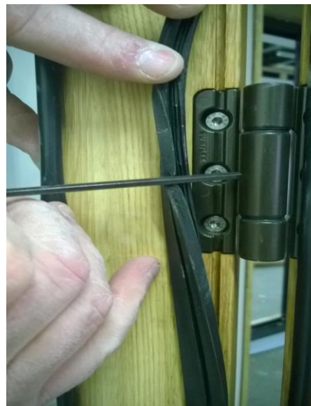
Photo 11 – Securing hinge pins
